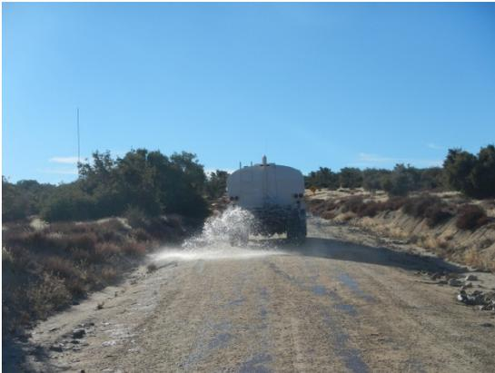
**Photo 3:** ECMs observed water trucks pre-watering access roads to minimize dust caused by moving vehicles and heavy equipment.
