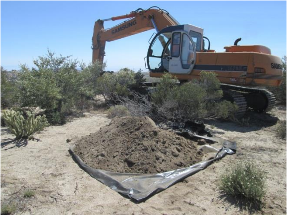
Photo 3: ECMs observed track hoes/excavators salvaging topsoil for restoration activities at the conclusion of geotechnical activities in accordance with the NTP conditions of approval.
