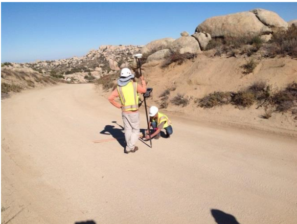
Photo 3: Survey crews staking road taper areas in accordance with MM BIO-1A.
