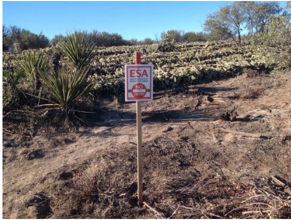
Photo 1: Salvaged cacti staged at laydown yard near Structure E2. ESA signs were installed to mark the area in accordance with Section 5.2.2.1 of the Habitat Restoration Plan (MM BIO-1D).
