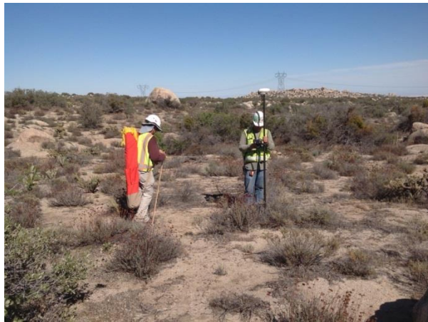
Photo 3: Survey crew staking the grading limits along the G String in accordance with MM BIO-1A.
