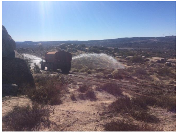
Photo 2: Water trucks observed applying water ahead of clearing activities in accordance with MM AIR-3.
