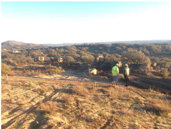
Photo 3: ECMs observed a Fire Patrol monitoring the clearing activities along the G line in accordance with MM FF-1.
