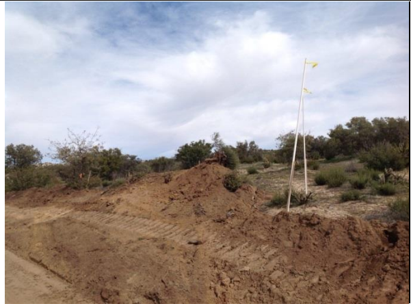
Photo 2: Contractor personnel added steel posts and PVC extensions where needed to give equipment operators greater visibility of limit of disturbance markers in response to the noncompliance event on February 9, 2017 (described in the caption of Photo 1).
