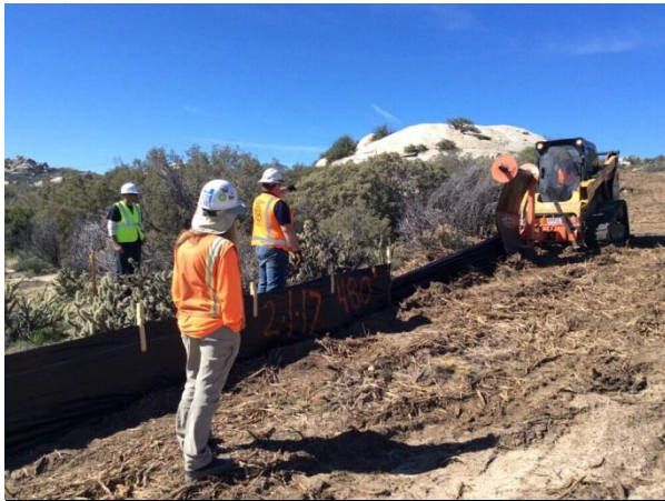
Photo 3: Archaeological and Native American monitors observed the installation of silt fence near site E13 in accordance with MMs CUL-1D and HYD-1.
