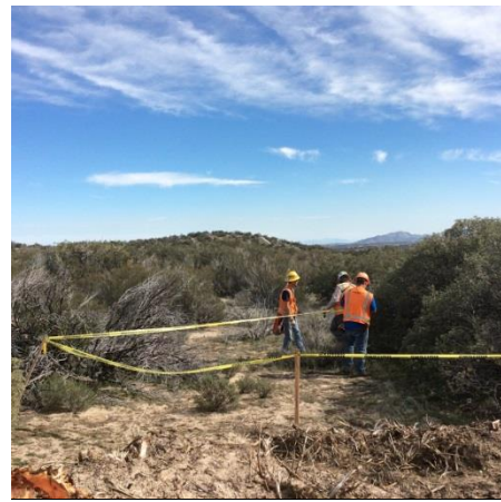
Photo 4: Crews observed verifying disturbance limit stake locations and installing yellow tape prior to the start of disturbance activities in accordance with the NTP issued February 1, 2017.
