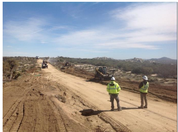
Photo 4: Biological, archaeological, and Native American monitors were present during road widening activities along McCain Valley Road in accordance with MM CUL-1D and BIO-1C. Water was applied regularly to reduce dust in accordance with the Dust Control Plan and MM AQ-1.
