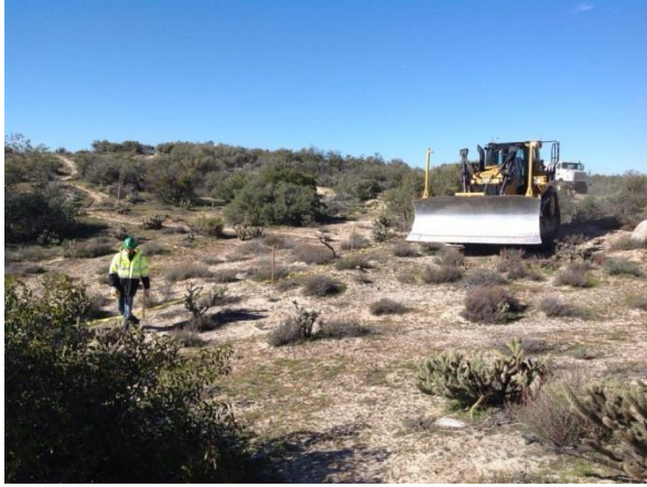
Photo 1: Spotters walked ahead of bulldozer operators who cleared large vegetation along the taped disturbance limits ahead of grubbing activities to help increase visibility for masticator operators in accordance with the February 1, 2017 NTP.
