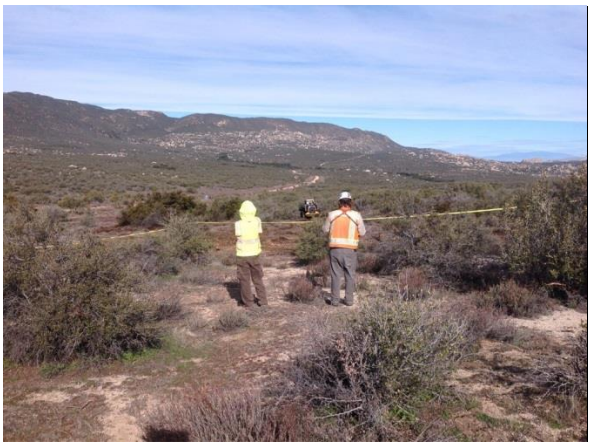
Photo 4: Biological monitors were present to observe grubbing activities in accordance with MM BIO-1C. All observed activities occurred within the disturbance limits in accordance with MM BIO-1A. Yellow tape was strung between disturbance limit stakes to increase visibility of limits for masticator operators in accordance with the NTP issued on February 1, 2017.
