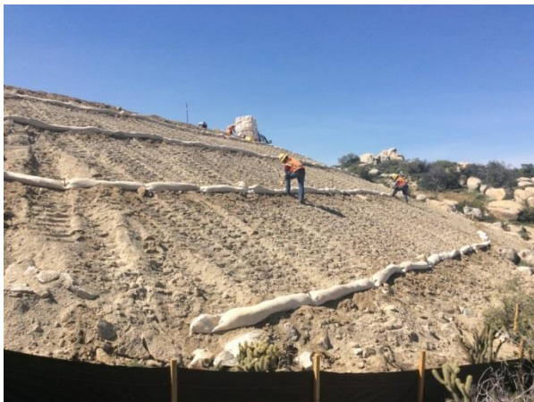
Photo 3: ECMs observed construction crews installing biodegradable and weed-free straw wattles at the H1 turbine pad in accordance with the SWPPP and per direction from the BLM, CDFW, and State Water Board.
