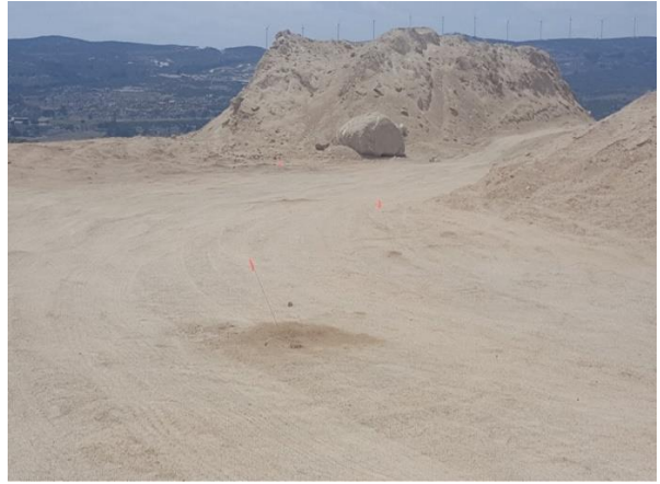
Photo 2: ECM's observed flagged, stained soil sites at turbine pad G15.
