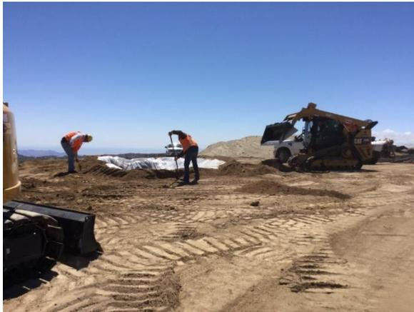
**Photo 3:** Construction crew installing concrete washout basin at turbine pad C3 in accordance with the project SWPPP.
