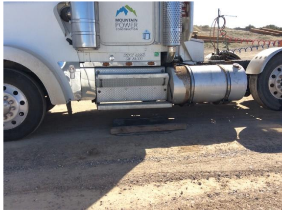
Photo 2: Drip pans were present under staged equipment in accordance with the SWPPP and MM HAZ-1A.
