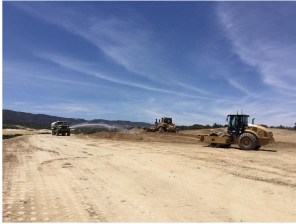
Photo 1: ECMs observed a water truck providing dust control during backfilling at turbine site E-3 in accordance with MM-AQ-1.
