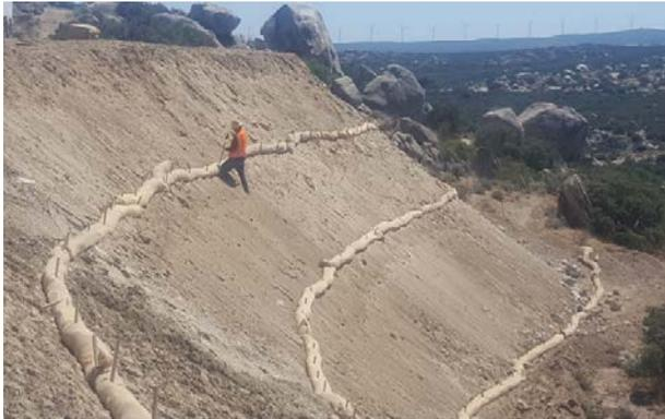
**Photo 1:** Straw wattle installation at turbine site E-10 in accordance with MM-HYD-1 and the site SWPPP.
