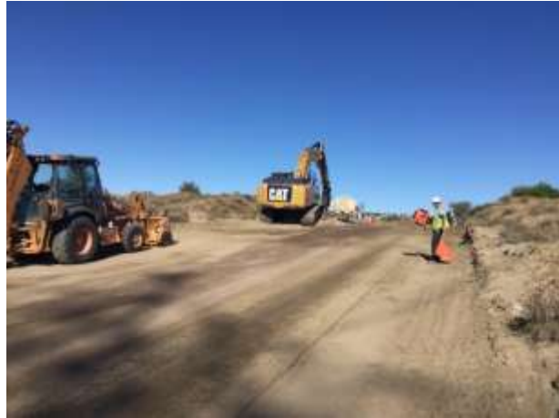
Photo 1: ECMs observed traffic flaggers present and signage posted at the entrance of McCain Valley Road in accordance with MM-TRA-1.
