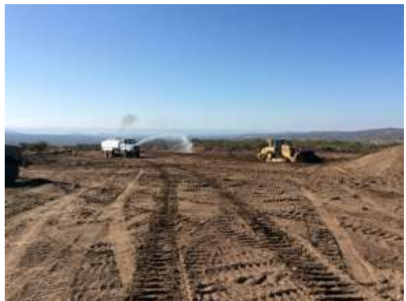
Photo 4: ECMs observed water tenders at turbine site B-5 during topsoil salvaging in accordance with the Dust Control Plan and MM-AQ-1.
