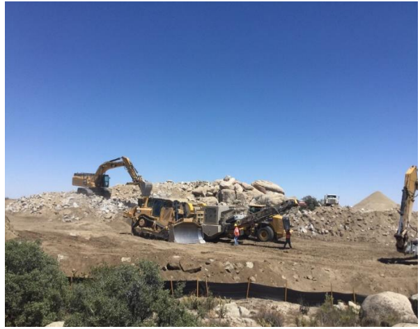
Photo 2: ECMs observed rock management at laydown yard #10, with water tender present in the background in accordance with MM-AQ-1 and MM-FF-1.
