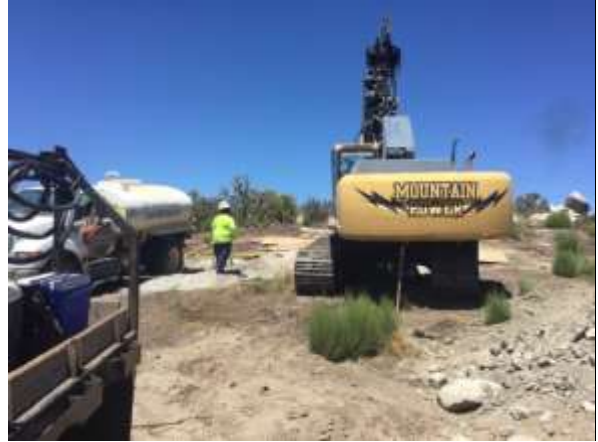
Photo 2: ECMs observed cultural monitors present during drilling activities at collector line site C57 in accordance with MM CUL-1D. A water truck was also present and work remained within the staked disturbance limits in accordance with MM AQ-1 and MM BIO-1A, respectively.
