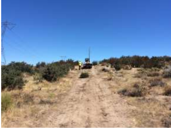
Photo 1: During this reporting period, ECMs observed spotters walking ahead of equipment installing stringing lead lines to ensure operators remained inside the marked limits of disturbance in accordance with MM BIO-1A.
