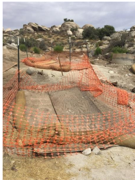
Photo 4: ECMs observed holes at collector pole 57 properly covered to prevent wildlife from becoming entrapped in accordance with MM BIO-7a.
