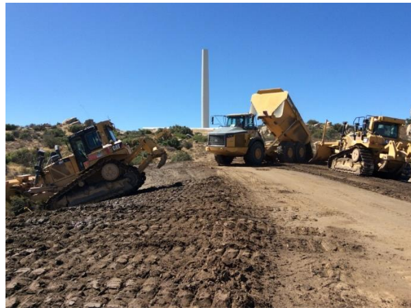
Photo 3: ECMs observe construction crews restoring temporary work areas by reclaiming topsoil to road shoulders, as pictured on the G-15 access road, pursuant to The Habitat Restoration Plan and MM BIO-1d.
