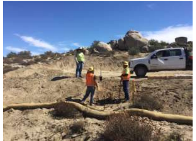
Photo 4: ECMs observed cultural and biological monitors present for erosion control maintenance and repairs in accordance with MM BIO-1D and MM CUL-1D.
