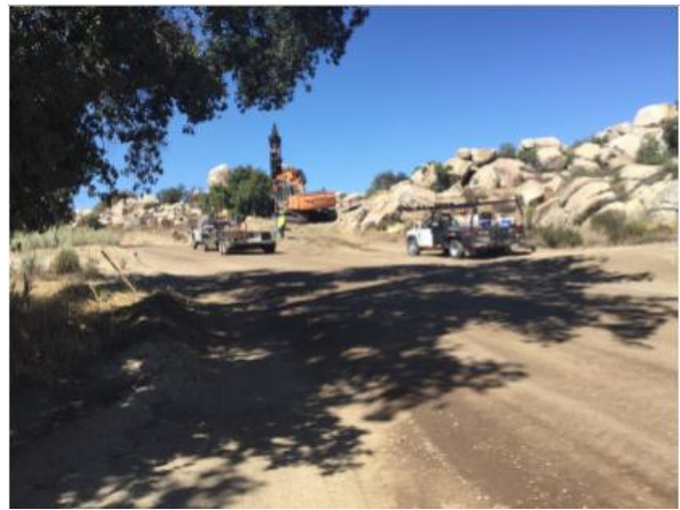
Photo 2: ECMs observed drilling at collector pole 60. A water truck was also present during drilling to minimize fire risk in accordance with the Fire Prevention and Protection Plan and MM FF-1.
