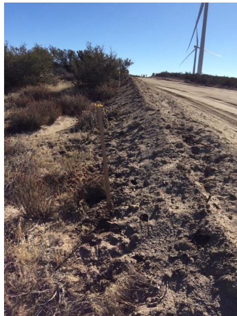
Photo 4: The protocols of Variance Request 006 were implemented to allow for disturbance beyond the staked limits of disturbance during road reclamation activities.
