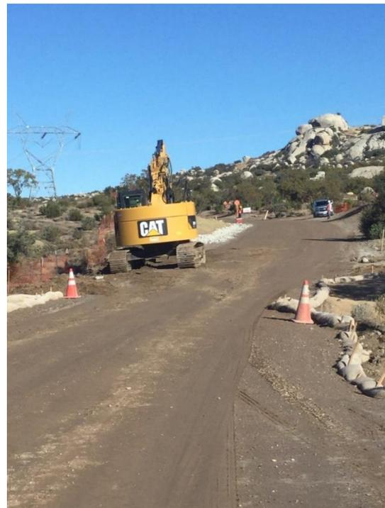
**Photo 4:** Culvert excavation and rip rap installation occurred along McCain Valley Road requiring implementation of Variance Request 006. This activity was monitored by biological and cultural monitors in accordance with the protocols of Variance Request 006.
