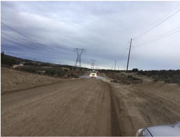
**Photo 1:** A water tender observed watering along McCain Valley Road in an effort to minimize dust, in accordance with the Dust Control Plan and MM AQ-1.
