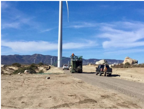
Photo 3: Hydro seeding observed along the G-line access road with a habitat restoration specialist present, in accordance with MM BIO-1c.
