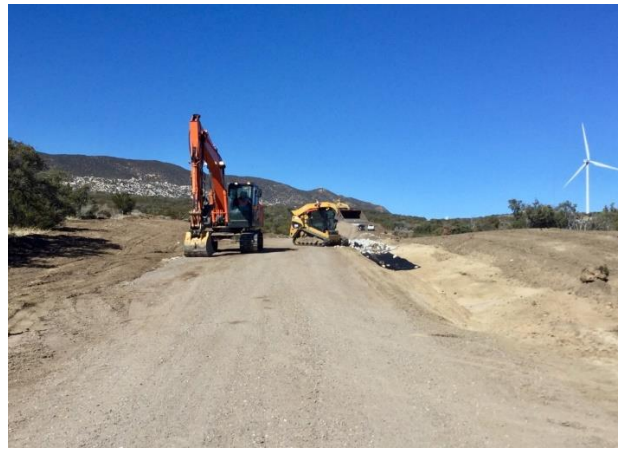
Photo 2: ECMs observed rock lined drainage swale installation along McCain Valley Road, near the A-line access road, per the site specific SWPPP and Grading Plans.
