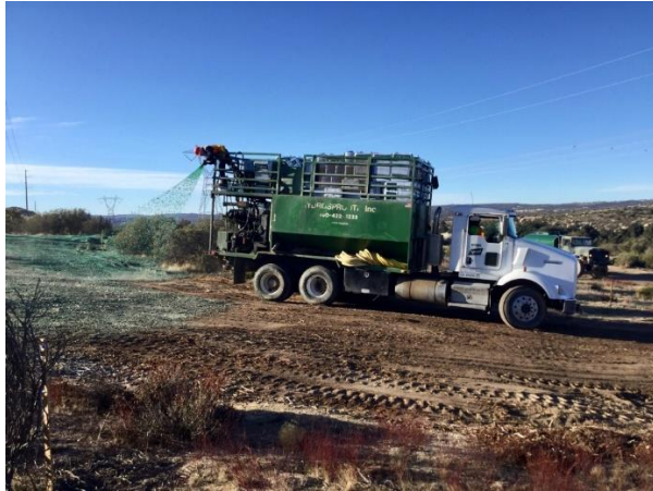
Photo 1: Hydro seeding along the Collector Pole Line in accordance to MM-BIO-1d and the Habitat Restoration Plan.
