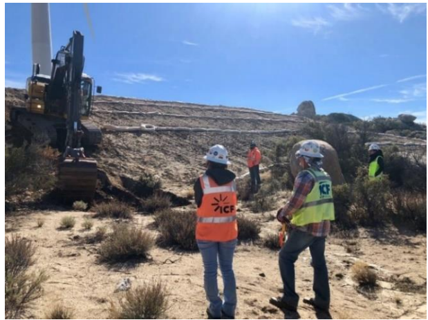
Photo 2: ECMs observed rock lined drainage swale installation along McCain Valley Road, near the A-line access road, per the site specific SWPPP and Grading Plans.
