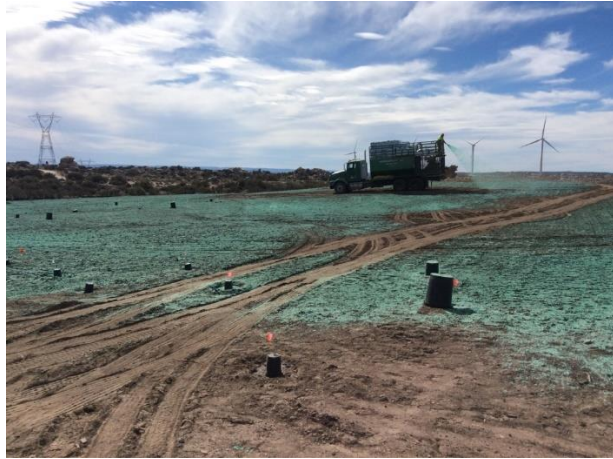
Photo 1: Hydro seeding occurred at laydown yard #11, in accordance with the Habitat Restoration Plan.
