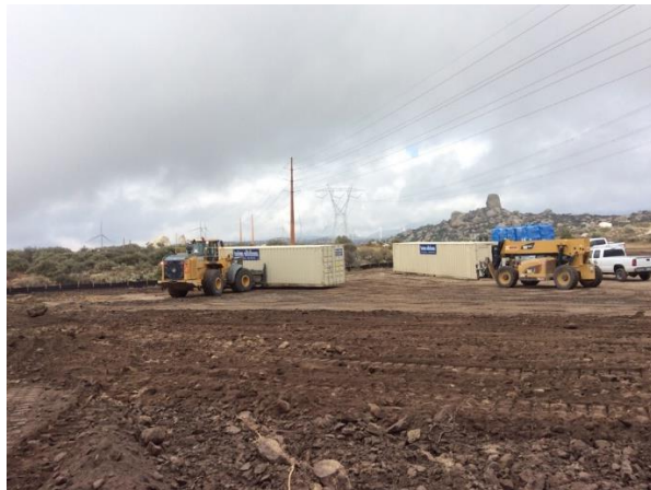
Photo 3: ECMs observed construction crews demobilizing laydown yard #9.
