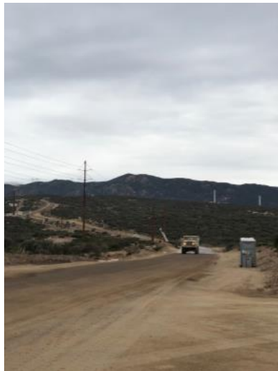
Photo 3: ECMs observed water trucks minimizing fugitive dust by applying water to access roads and other active work areas, in accordance with MM AQ-1.
